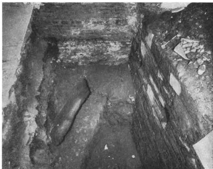
Fig. 70 — S. Lorenzo f.l.m. Excavations 1947-49. South aisle, wall D_{4-6} looking south (Photo: Sansaini).
